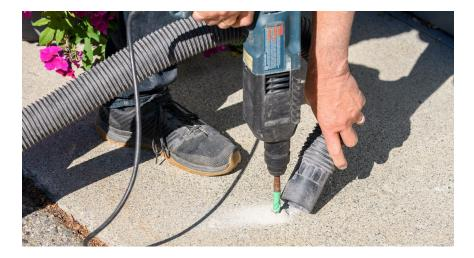
Hammer the concrete anchors into the clean drilled holes so they are slightly below flush with the surface. This is easiest with a sacrificial bolt.
