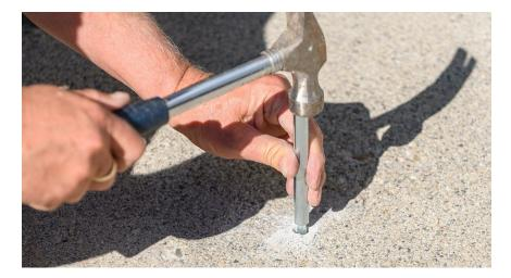
Position the bench on the concrete pad by lifting it in place. Line up the holes and ensure the anchors remain free of any debris.
