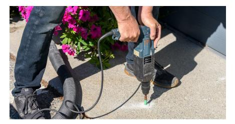
Vacuum (or blow) the drilling dust and debris to leave a clean hole. A screwdriver can be useful to loosen any debris in the hole.
