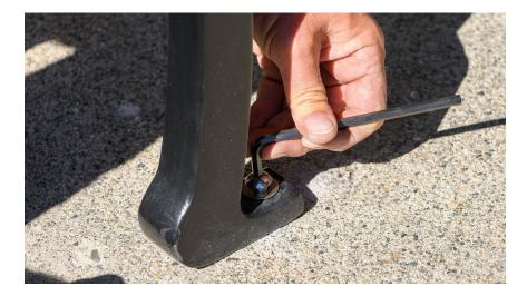
Optional. For theft resistance, fill in the bolt heads with silicone and paint the tops of the fasteners with a paint pen to match the colour of the frame.
