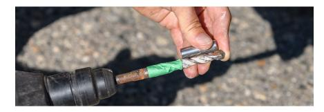
Drill all holes to the depth indicated by the tape or marker applied to the drill in step 4. Holes must be vertical to properly anchor the bench.
